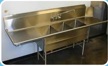
Dishwashing and or food preparation sinks are required to have an indirect connection to the sewer to prevent sewage from backing up into them.
